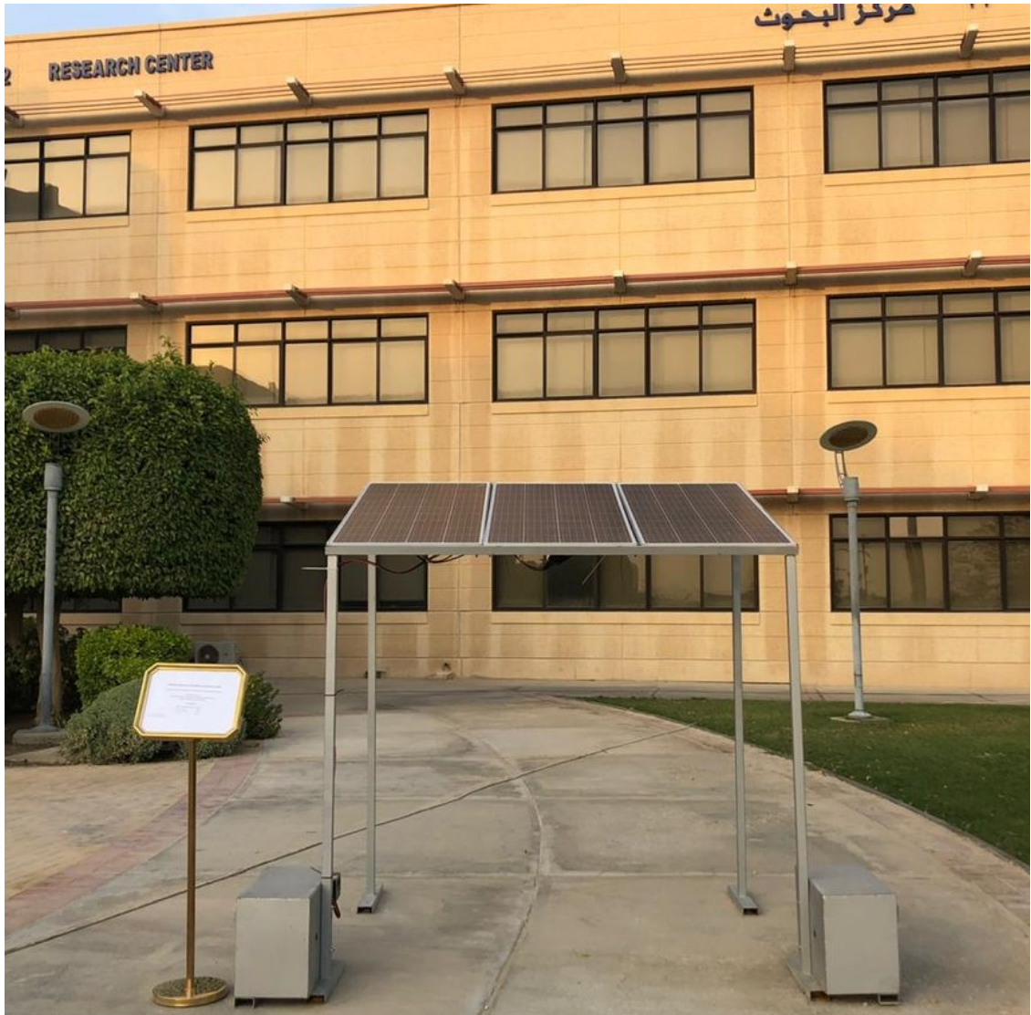
Figure 3.3: Implemented solar carport.
