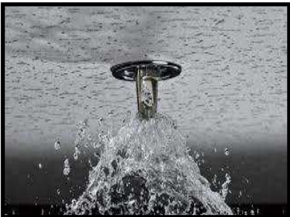
Figure 3.9 Sprinkler in operation
