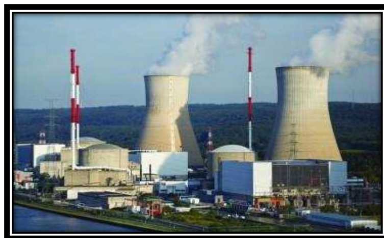
Figure 1.3 Electric power plant cooling tower
