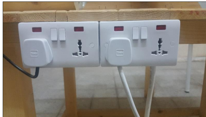
Figure (3.3) Electrical cable and wires
