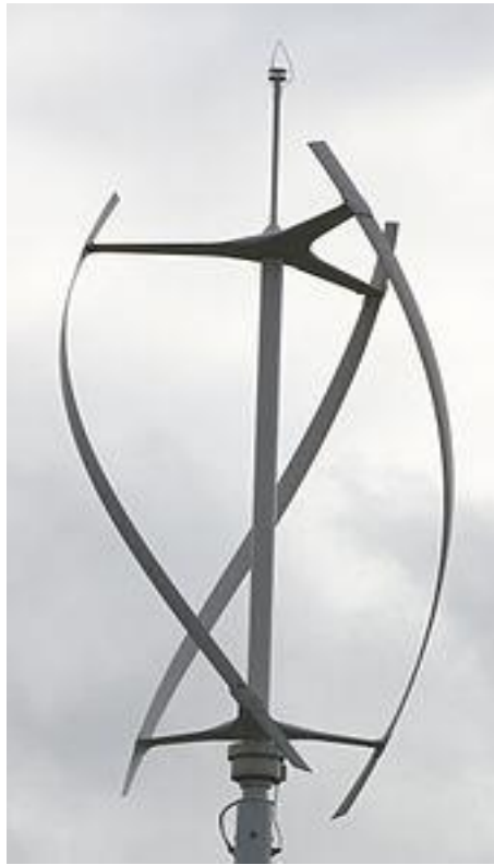
Figure 3.2 Gorlov Turbine
