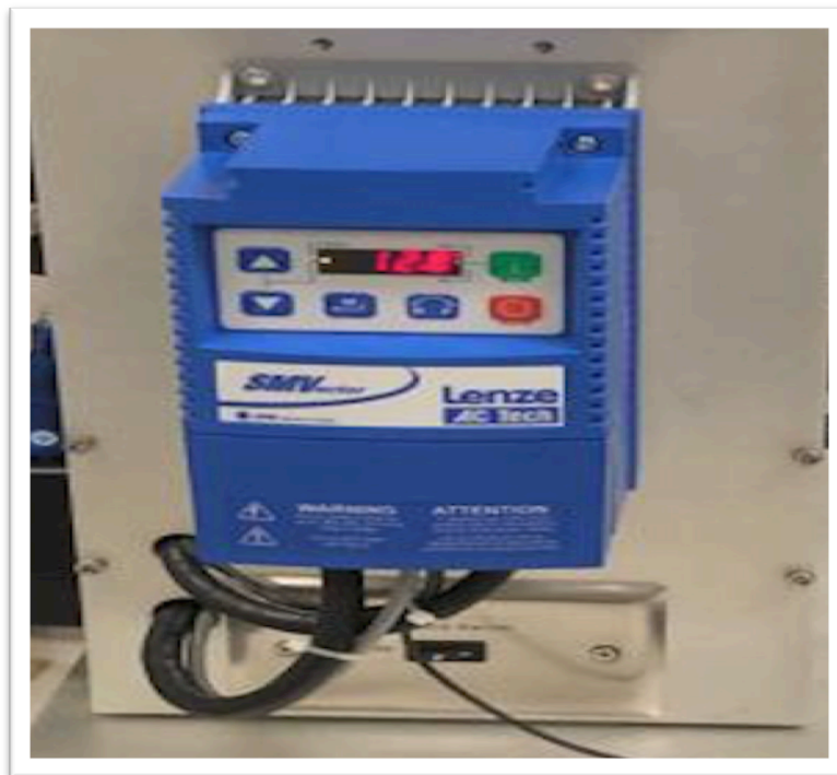
Figure 3.2.3.3a: Variable frequency drives
