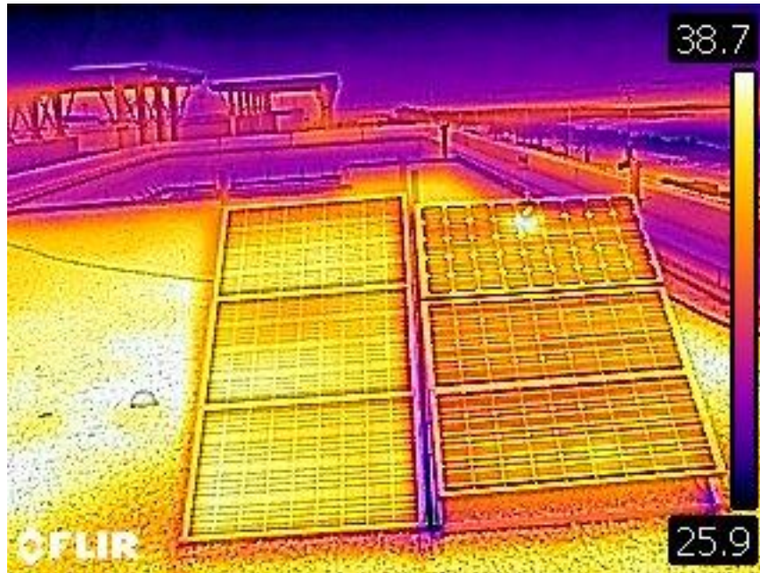
Figure 10b Normal PV Panel
