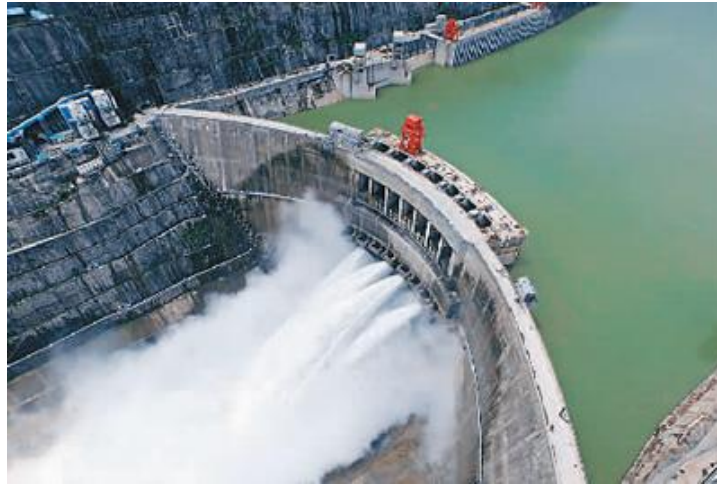
Figure 2: Hydroelectric Power plant
