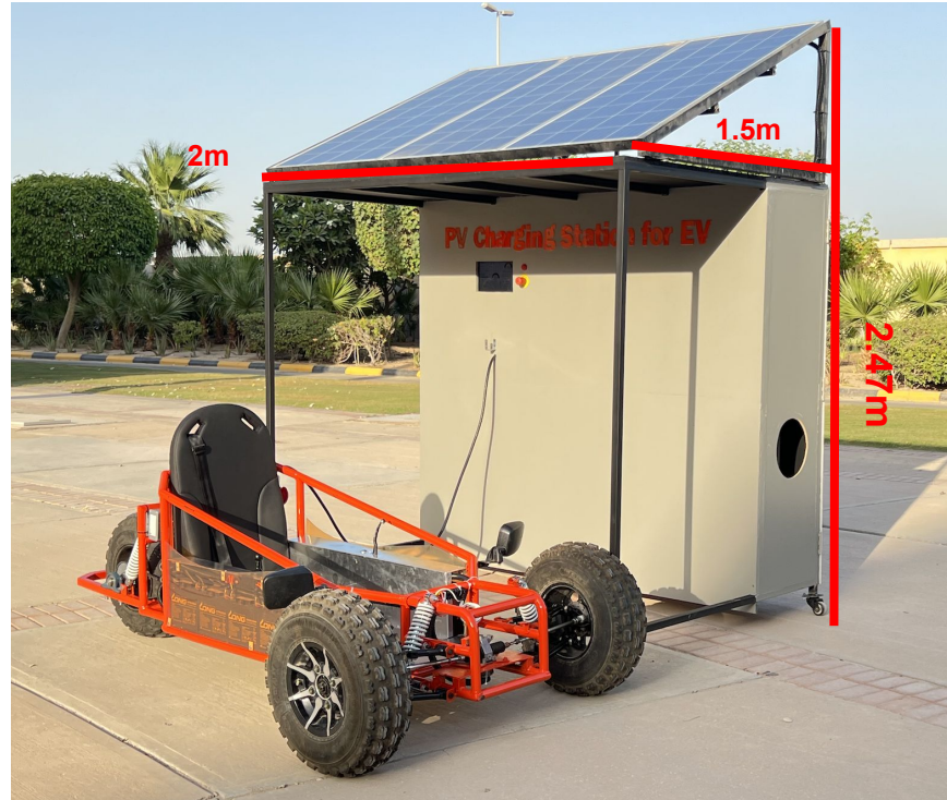
EV charging station
