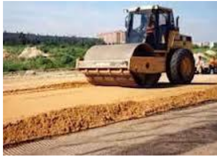
Figure 5.2. Mechanical compaction (photo 1, from internet)
