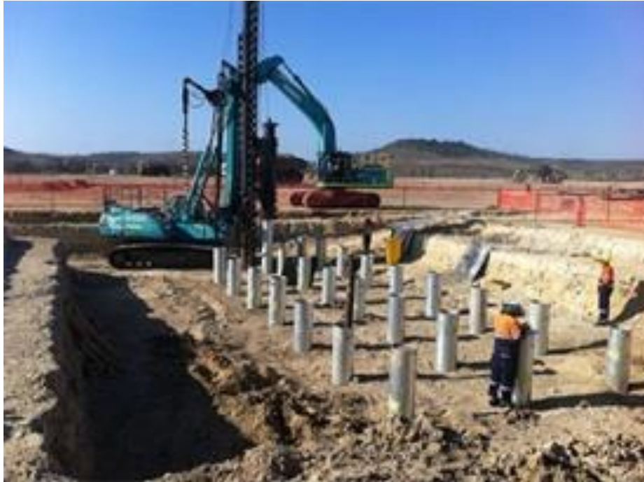
Figure 5.5. Deep foundation (driven piles, from internet)
