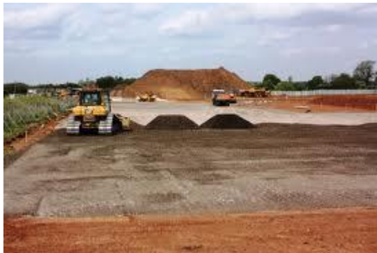
Figure 5.3. Mechanical compaction (photo 2, from internet)
