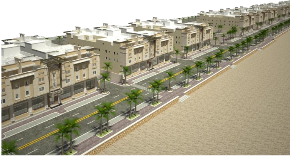
Figure 2.3. Overview of the complex (photo 2)
