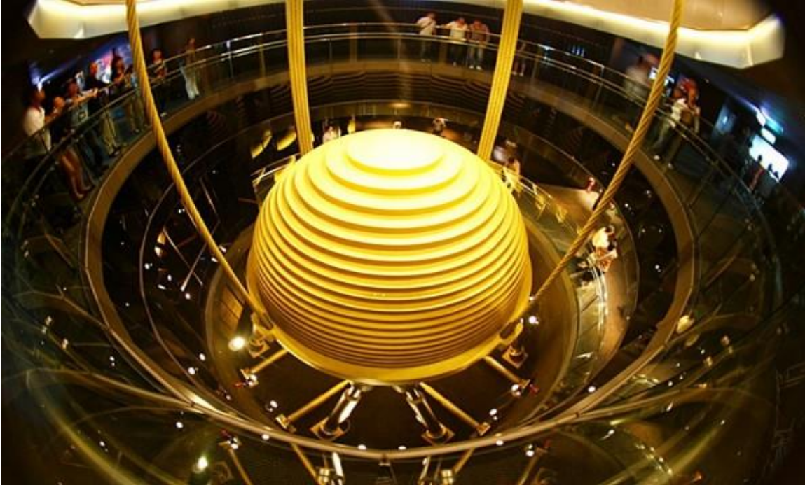
Figure 5 Example on passive damper system (8)
