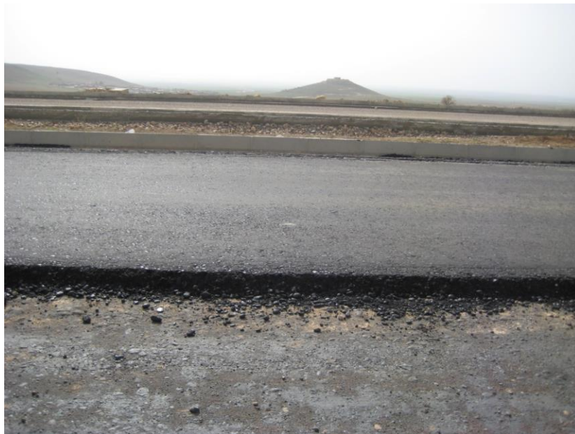
Figure 5.14. Example of pavement construction (photo 2)
