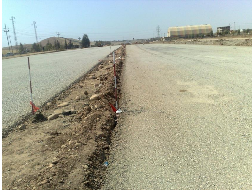
Figure 5.13. Example of pavement construction (photo 1)
