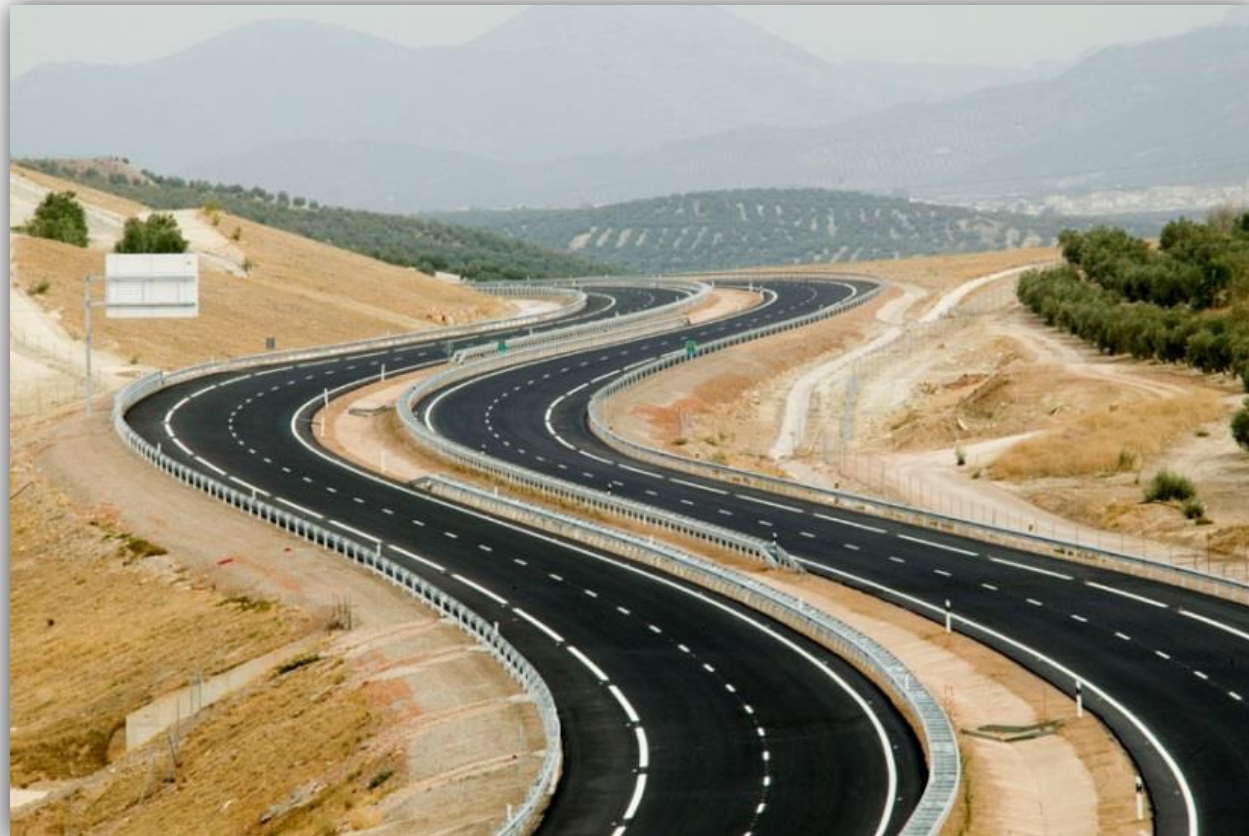
Figure [11]-Horizontal alignment example
