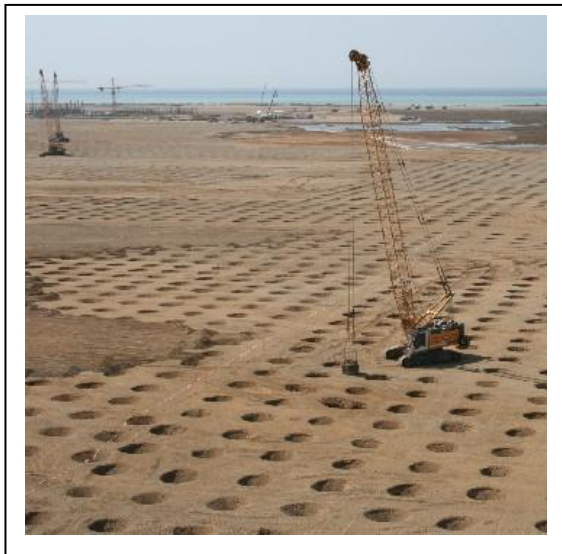
Figure 5.2. Process of dynamic compaction (#1)
