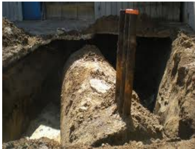
Figure 1 : Underground Storage Tank
